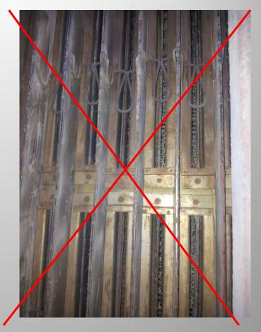
Low pressure loss / high regeneration efficiency by open bag supporting
